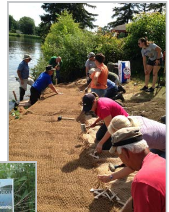
Participants in a Certified Natural Shoreline Professionals training class repair an eroding bank on Maple Lake in Paw Paw, July 2015.
